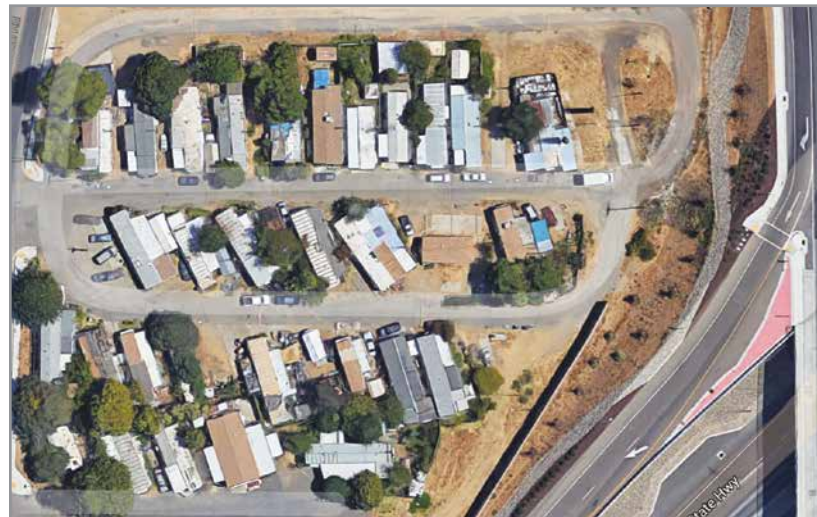
Figure 3 Aerial View of the Mobile Home Park
