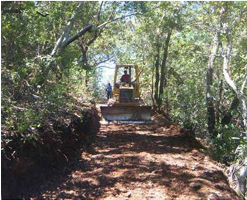
Figure 5 Bulldozer Clearing and Grading for Adventure Park Roadway
