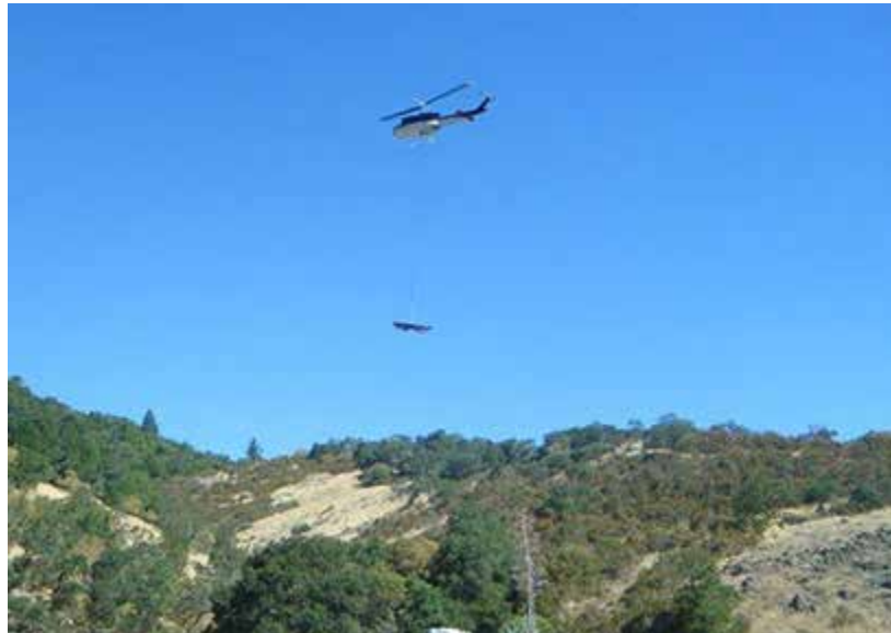
Figure 4 Helicopter Transporting Materials During Zip Line Construction
