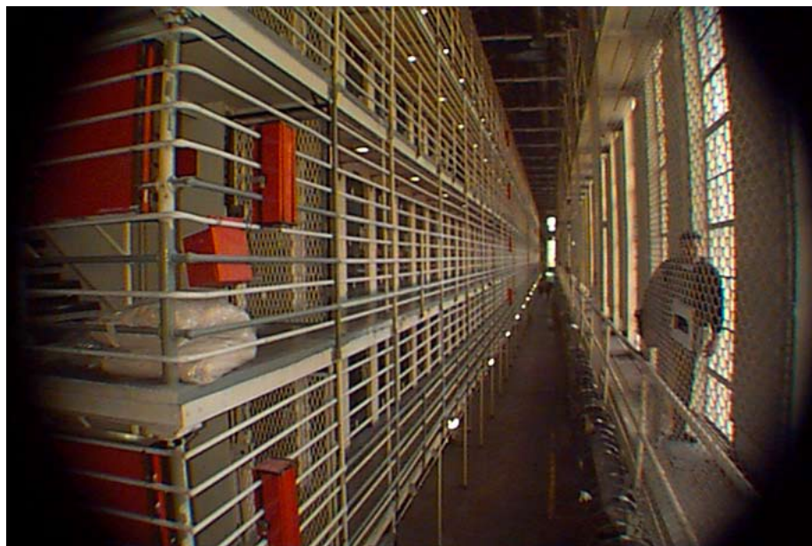
View Inside the East Block Facility
